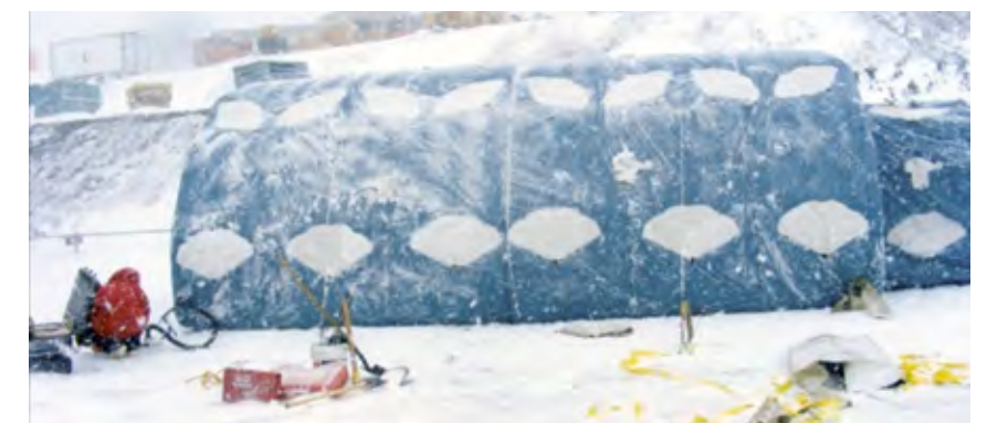
Complete setup took an average of 50 minutes, while inflation and deflation steps took up only 6 of those 50 minutes
