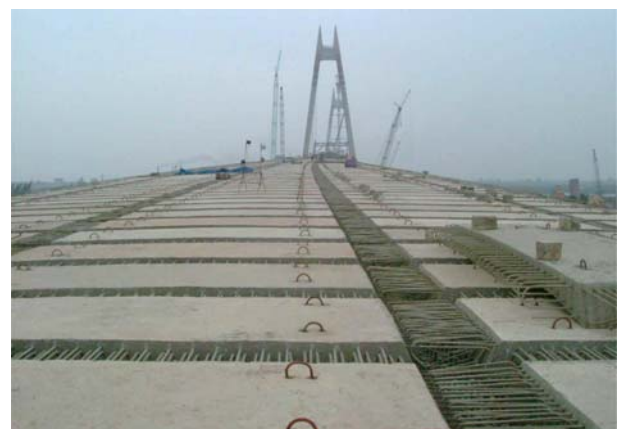
Fig. 22 Installation work of pre-cast concrete deck slab
