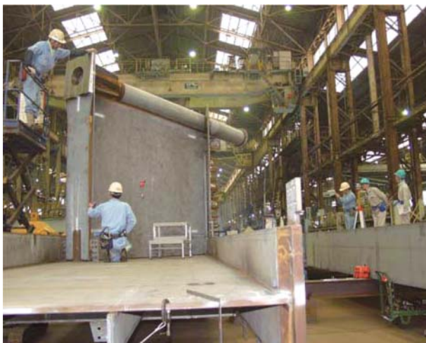
Fig. 14 Temporary assembly of main girder and anchor
