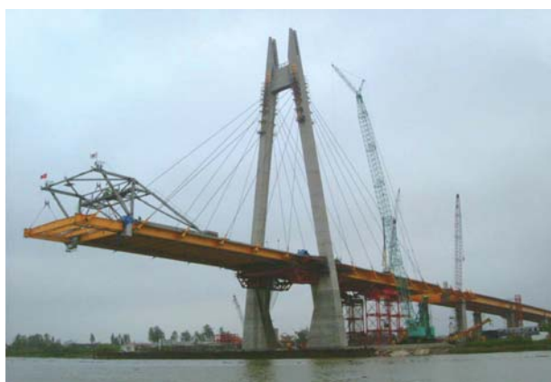
Fig. 21 Lifting method of steel girder for main span
