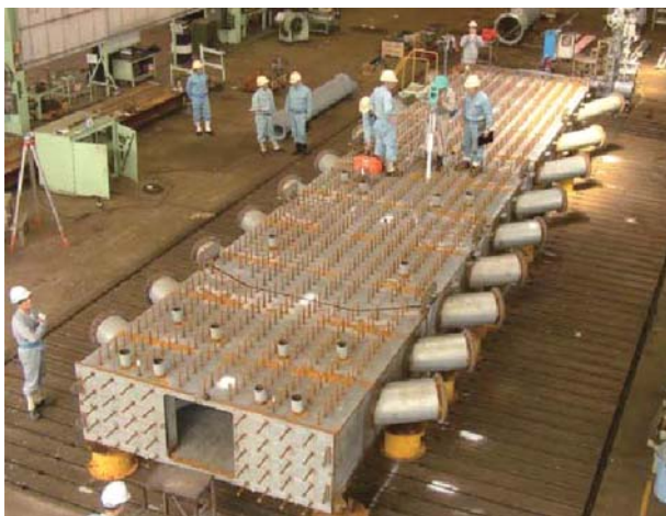
Fig. 13 Temporary assembly of anchor box
