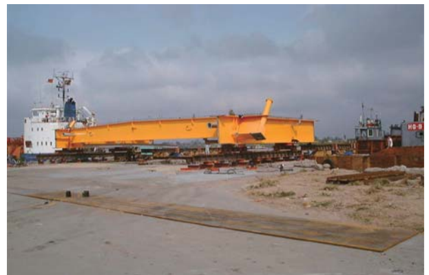
Fig. 20 Transferring procedure of steel segment onto barge
