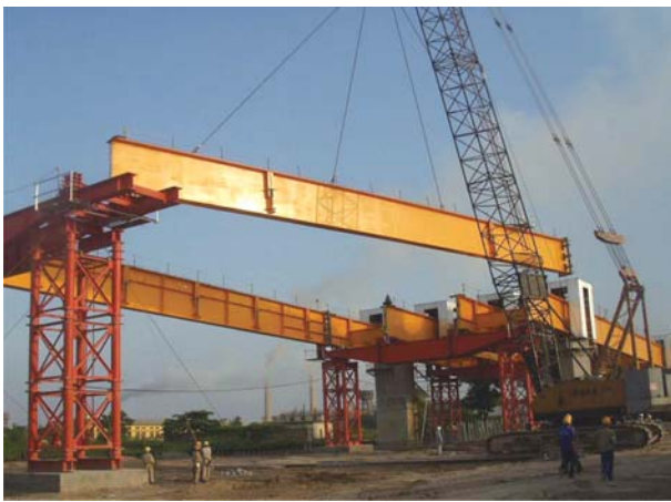
Fig. 18 Erection of steel girder for approach span
