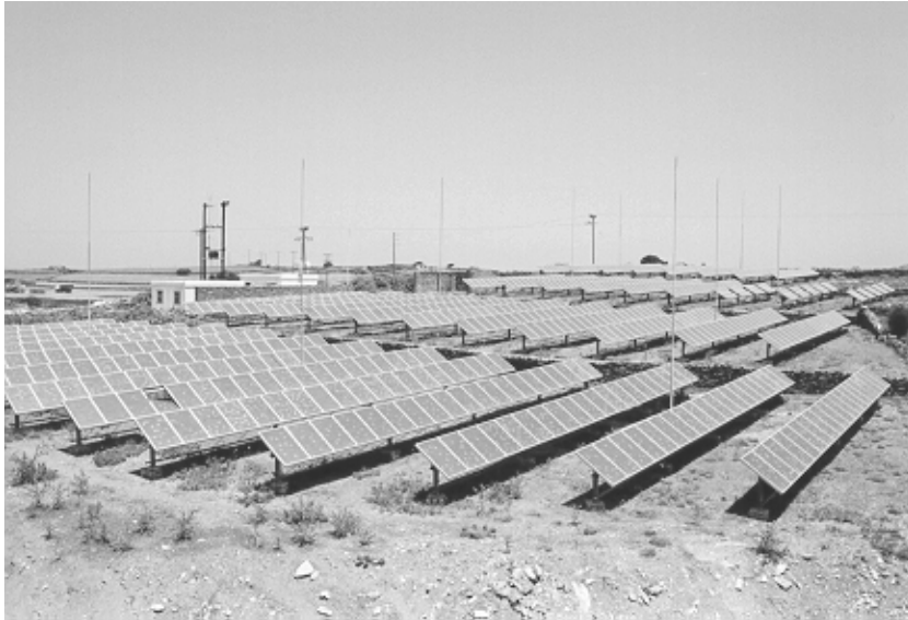
Abb. 2: Photovoltaik-Anlage, 100 kW
