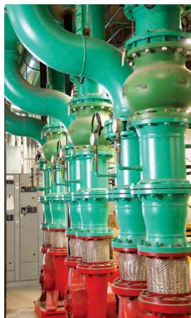
Chilled water pipes in the NCCS's mechanical room provide cooling to the center's machines.
