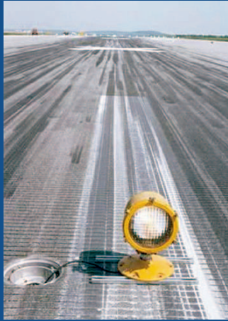
Damage caused by wheels
