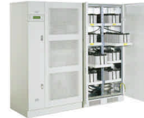
Uninterruptible Power Supplies
