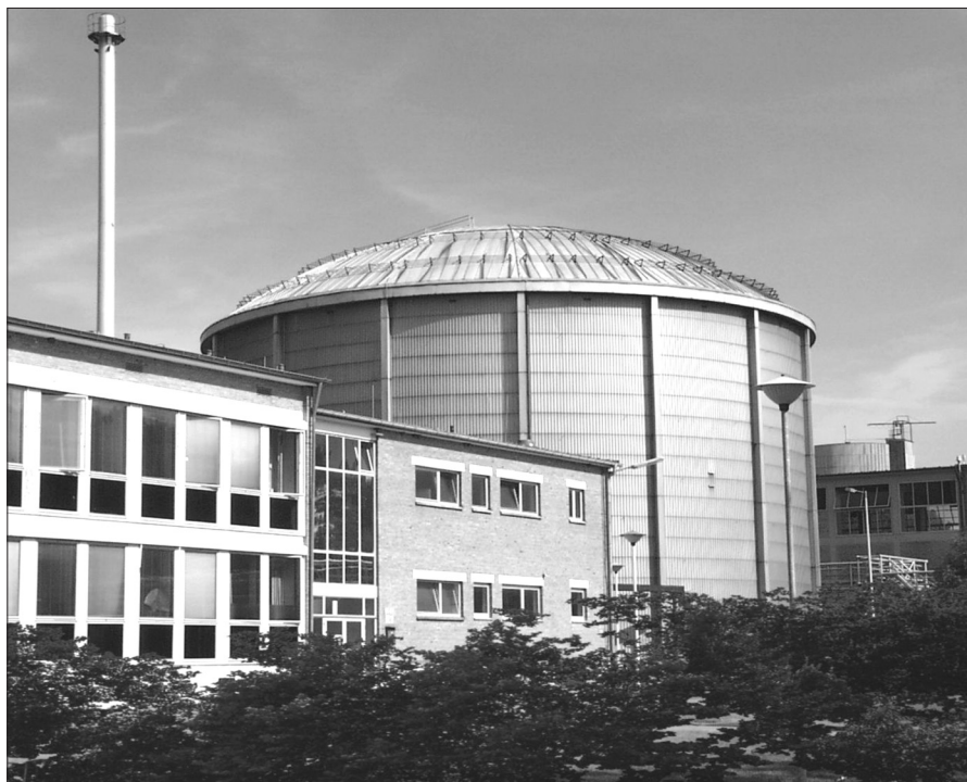
Fig. 1. Research reactor FRJ-2 (23 MW th ) at Forschungszentrum Jülich , Germany.
