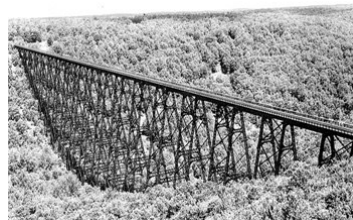
Kinsua viaduc, Pennsylvanie, 1900, Haut 92m, Long 625m
