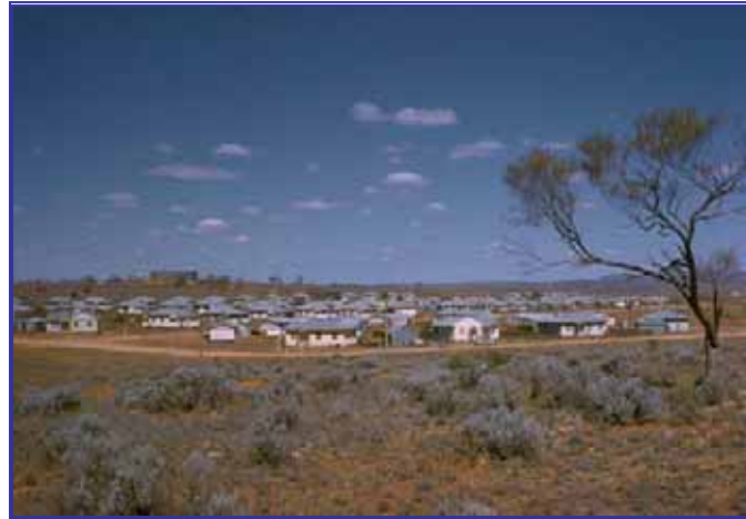
Fig. 19 Radium Hill township looking easterly towards the water tank on the hill, in the 1950s. (Source: PIRSA T022449)
