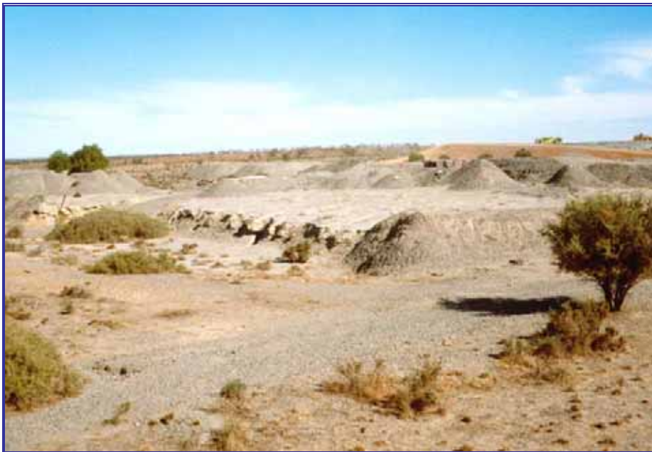
Fig. 30 ‘Kevin Carter’ tailings pile, prior to covering, 1981. (Source PIRSA 049698)
