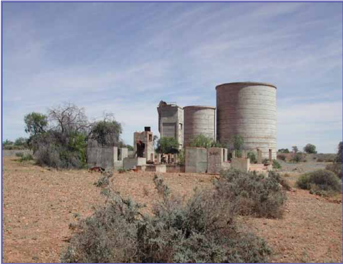
Fig. 12 Northerly view of the Radium Hill mill area and ore bins in 2004. (Source: PIRSA 049701)
