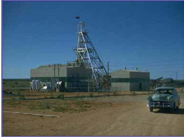
Fig. 10 Radium Hill Mine headframe, winding house (right) and compressor house (left); the ore hoppers are located directly behind (not visible) the hoist; 1954. (Source: PIRSA T000002)
