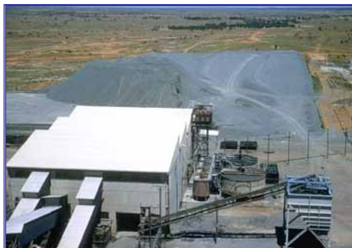
Fig. 27 Portion of the waste-rock dump area and heavy-media separation piles at Radium Hill in the 1950s. The large pile is often referred to as Mt Nelson. (Source: PIRSA T004524)
