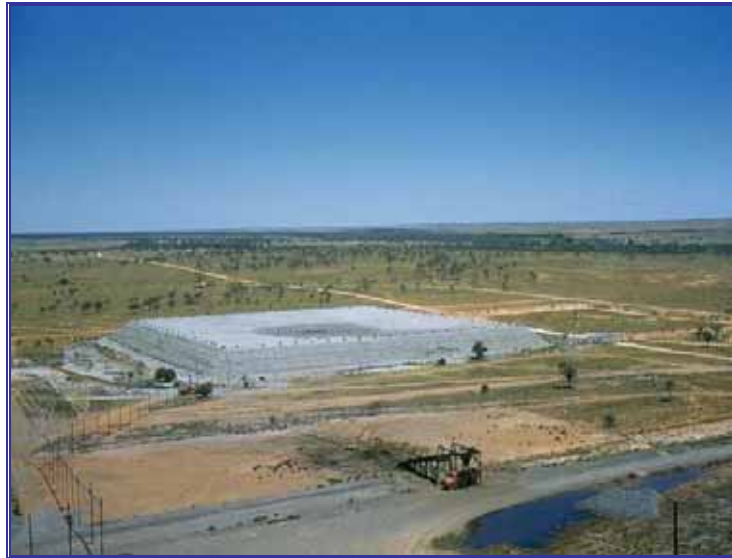
Fig. 15 Radium Hill Mine tailings impoundment, viewed southwesterly from the top of the headframe, in the 1950s. Note the spillage of material to the left. (Source: PIRSA T004525)
