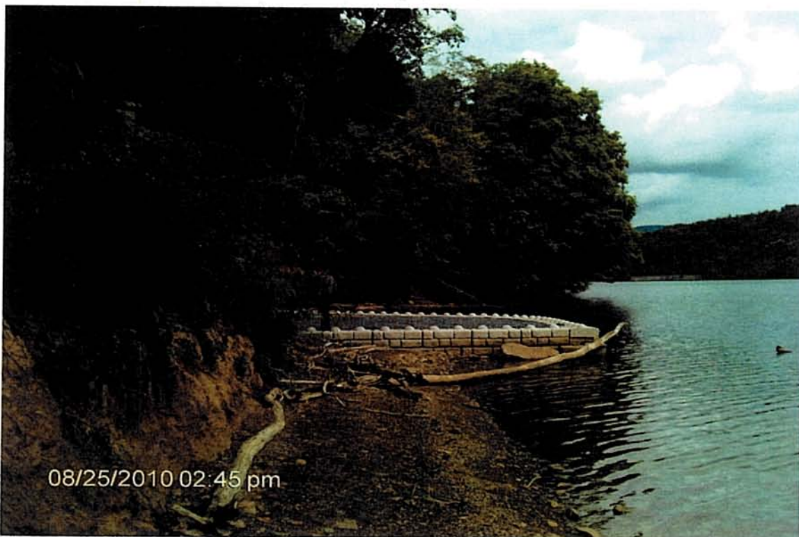
Photo 2: Sea Wall Facing Downstream on Cheat Lake
