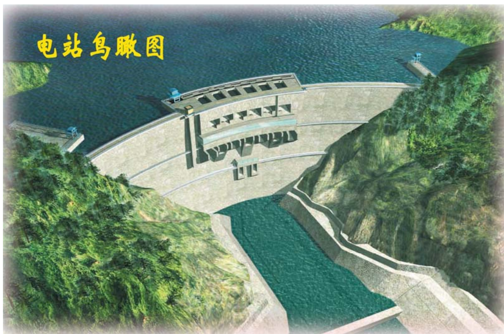
Bird's view of Goupitan Hydropower Project
