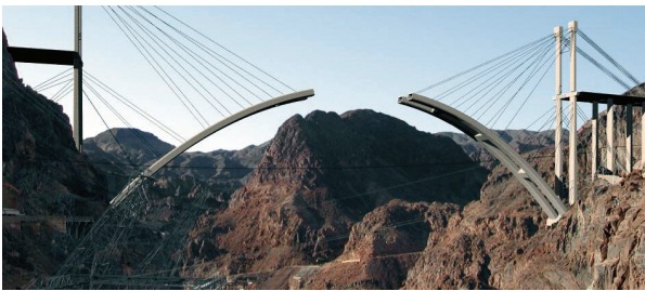
Fig. 5 - Stayed Arch Erection
