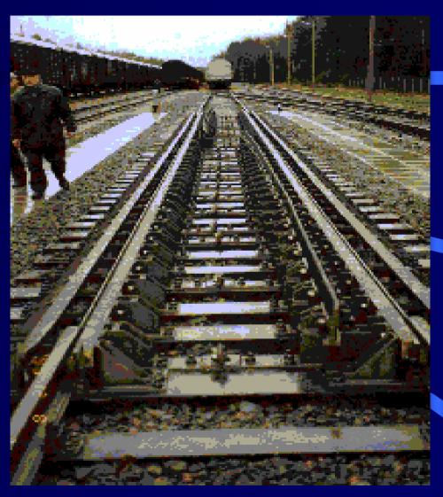
Track gauge changing facility (TSP) at the 1435/1520 mm interface at Mockava station (LG)
