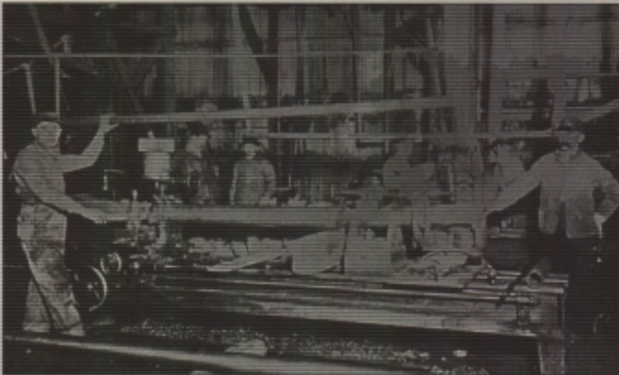
Water-powered machine shop in full operation.
