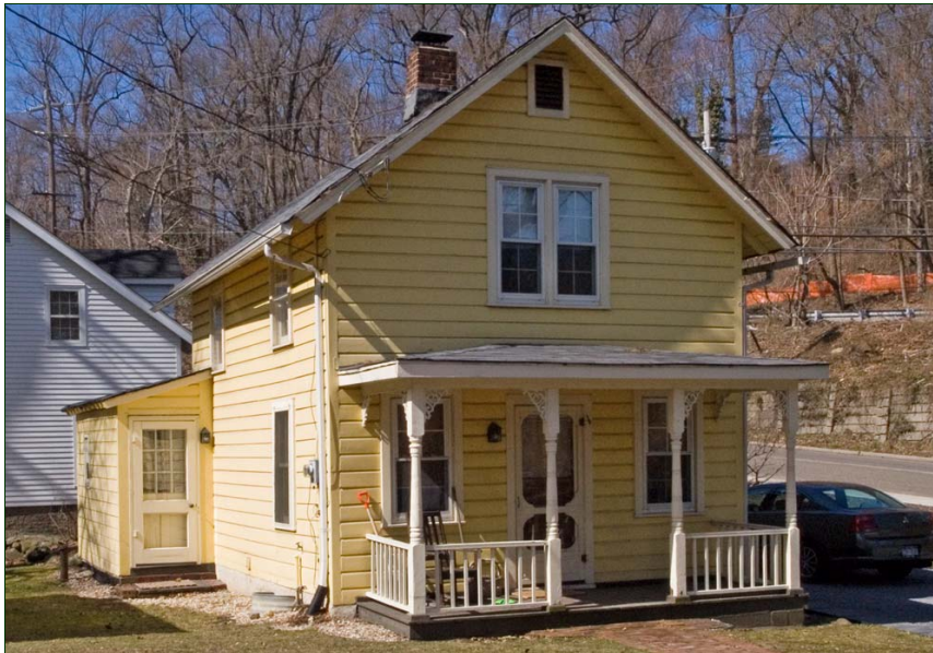
The Estelle Seaman Cottage has overhanging eaves and a spindlework porch.
