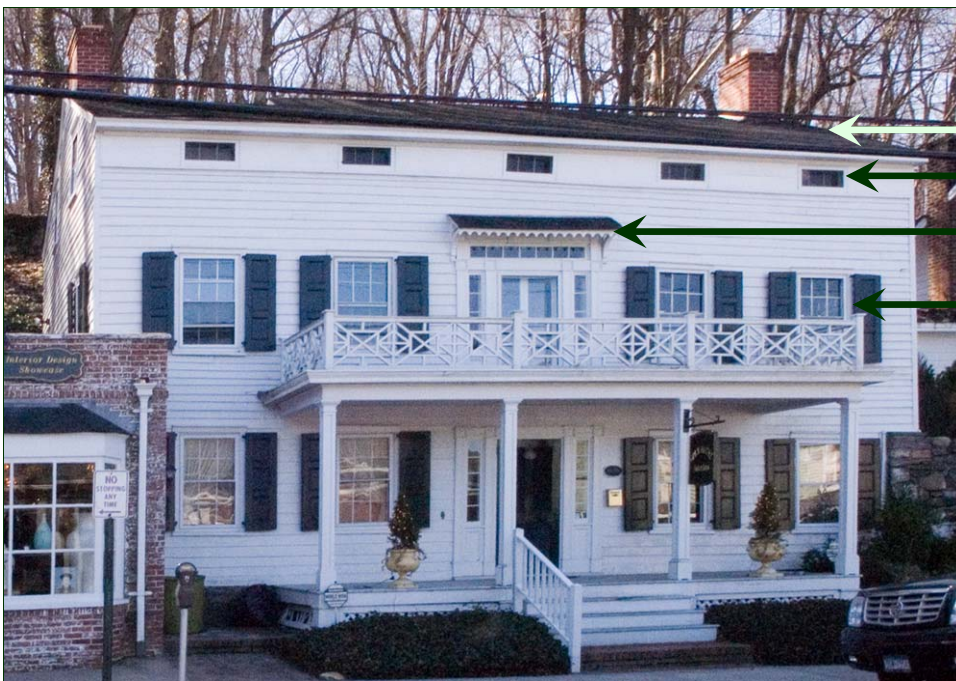
The c. 1830 George Allen House typifies the Greek Revival style with its symmetrical façade, small windows at the wide roof cornice board, and narrow transom windows and sidelights at doors.
