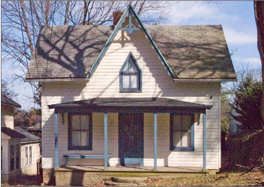
This cottage's vernacular Gothic detailing includes a steeply pitched roof and pointed arch window.
