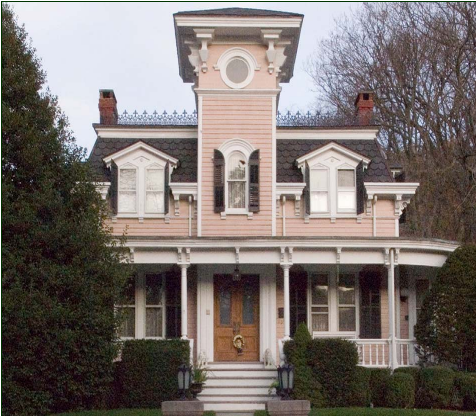
This Second Empire house features a Mansard roof with projecting eaves featuring heavy brackets.
