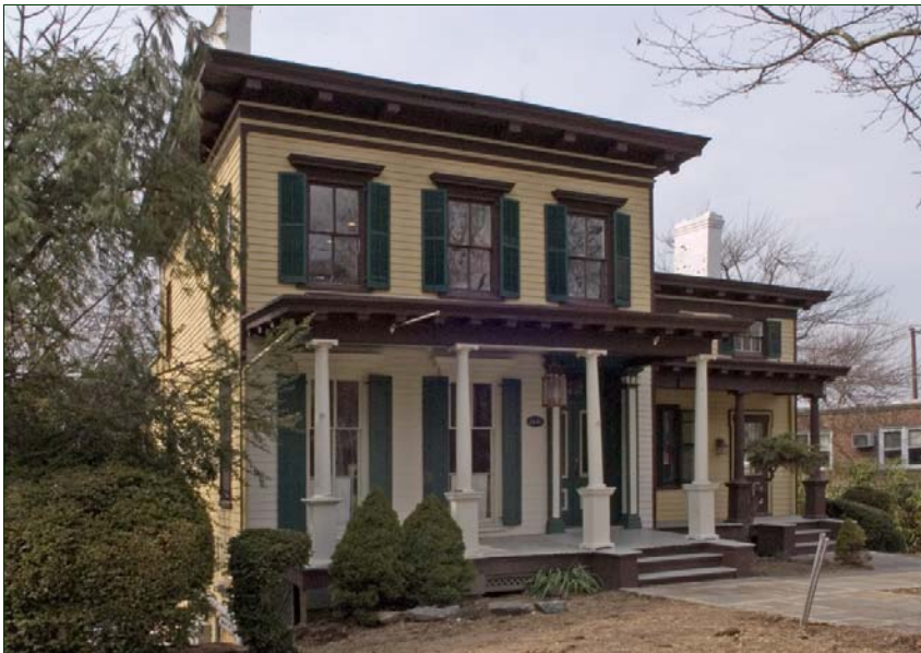
The c. 1858 Willet Titus House has elaborate wood molding at the windows and cornices.
