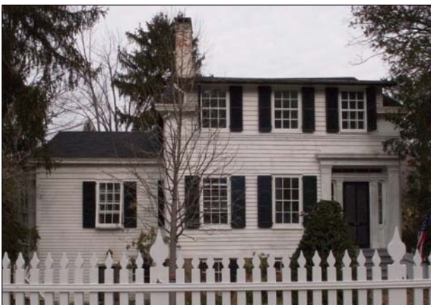
The Obadiab Washington Valentine House c. 1835 features classical pilasters and a prominent cornice at the front entry. The paneled door has a narrow transom and sidelights. A shed roof dormer was added in about 1910 along most of the principal façade allowing for taller windows at the second floor.
