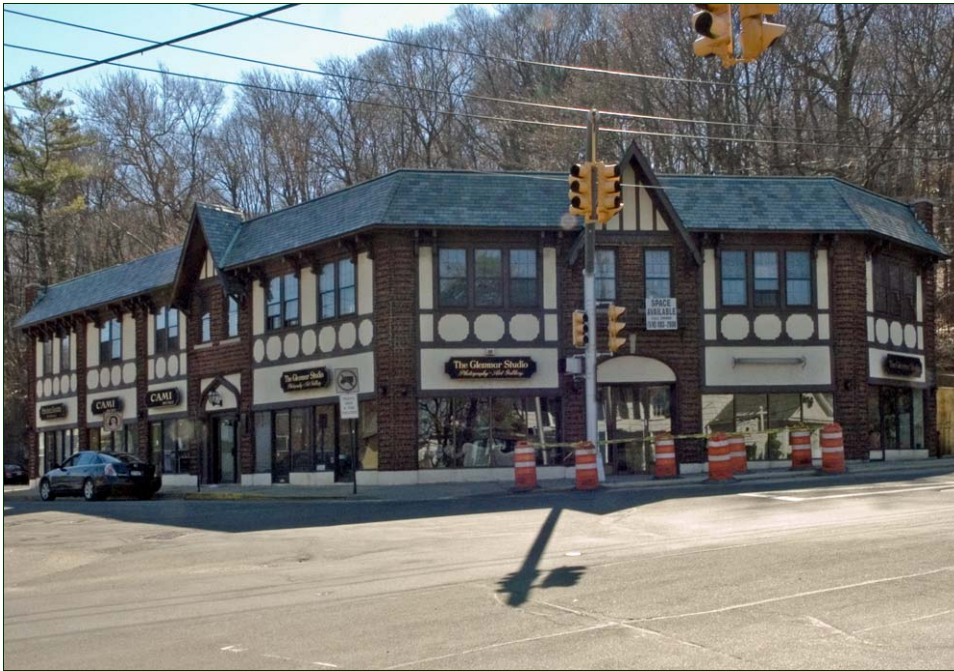
This Tudor Revival Building features elaborate half-timbering below the second floor windows.
