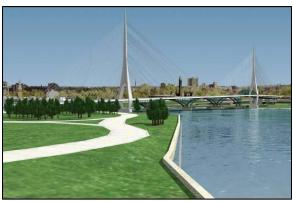
173 meters (567 feet). The cables connect to the outside edges of the roadway and run to the outside face of the towers near the base, which transition to the central spindle near the top.
