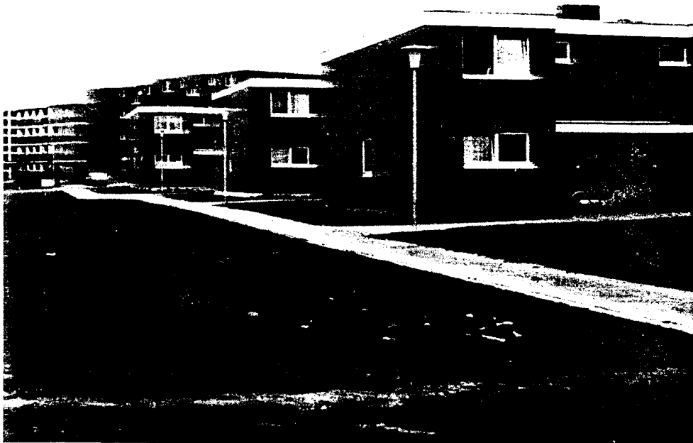
Garteler Weg Housing Area
