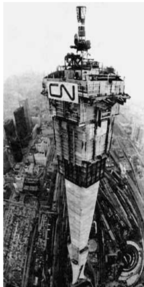
Figure 3: CN Tower under construction in 1976
