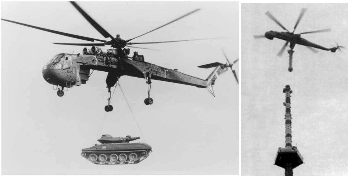
Figure 9: CH-54 Tarhe giant Sikorsky helicopter used to lift the 44 pieces of the antenna into place 5
