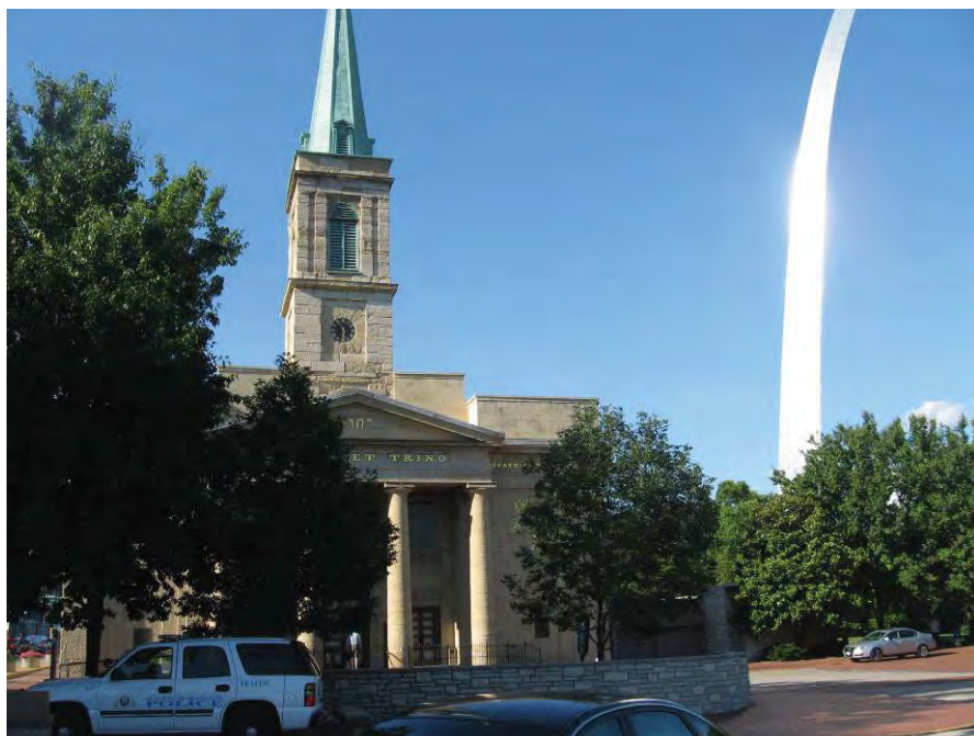
The Old Cathedral as viewed from the south.
