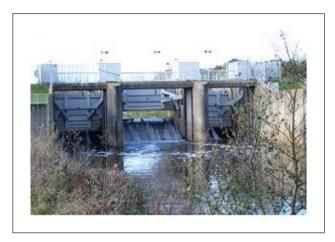
The storage area behind the Leigh Barrier is 278 hectares (686 acres) (that is about 255 football pitches), and when the land is flooded it can hold 5,580 million litres of water (1,230 million gallons). Before the barrier was constructed Tonbridge would regularly flood – the last serious floods being in 1968. See www.environment-agency.gov.uk for more information about the barrier.
