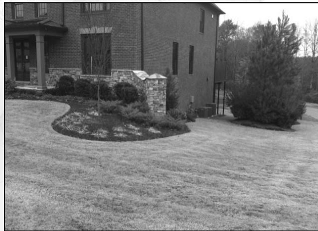
The grading of your homesite is meant to protect your foundation from water run-off and may include such features as retaining walls.
