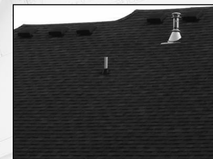
For shingles to lie down properly, they need to be in the warm sun so their adhesive mastic will heat and keep the layers sealed.
