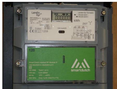
Figure 22: Smart Dutch RF module in a Landis+Gyr meter at Delta
