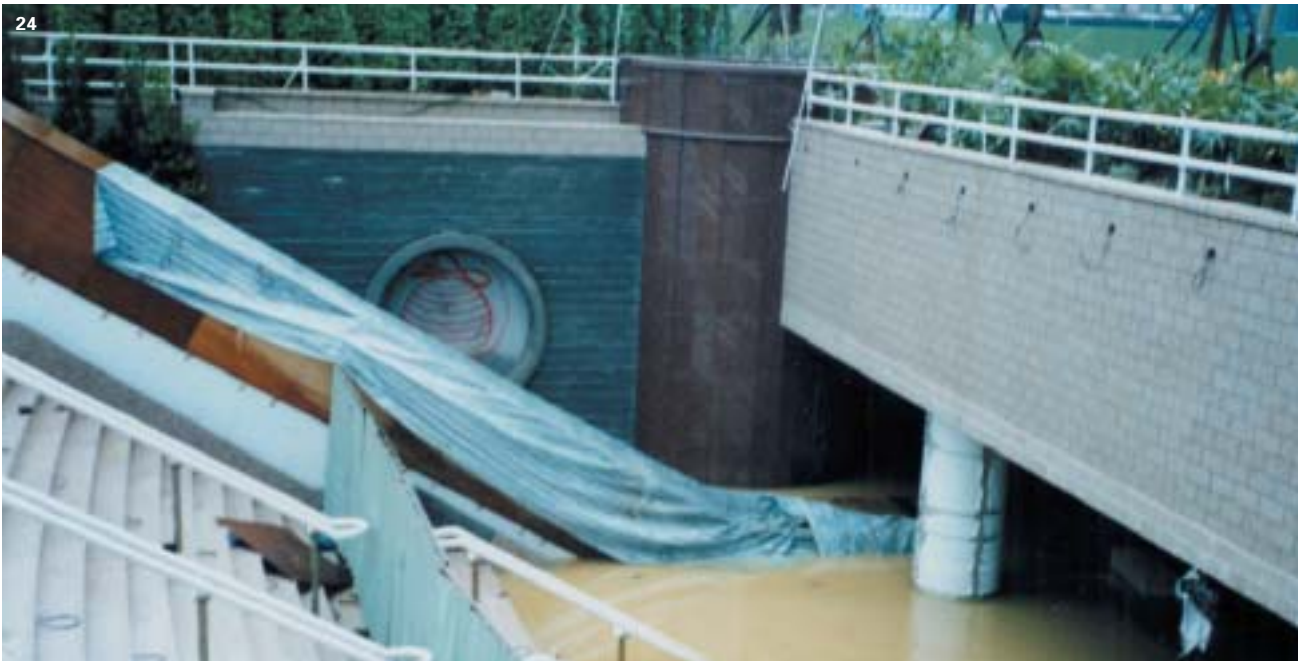
An underground station in Taipei. Power failures and the insufficient capacity of the pumps that had been installed led to some underground stations being completely flooded. Train services were limited for weeks on end.
