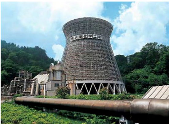
Fig. 8.47 Dry steam geothermal power plants (top left to bottom right): Lardarello, Italy; The Geysers, USA; Matsukawa, Japan; Kamojang, Indonesia (source: [2001Ano d ; 2003Sat; 2004Lun a ; 2004Wor]).
