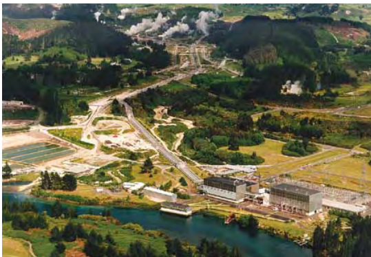
Fig. 8.51 Wet steam geothermal power plants with triple and dual flash cycles (left to right): Wairakei, New Zealand (with prawn pond in foreground) and Imperial Valley, USA, respectively (source: [2001Ano d ; 2002Ano]).
