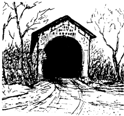
Moscow Covered Bridge
