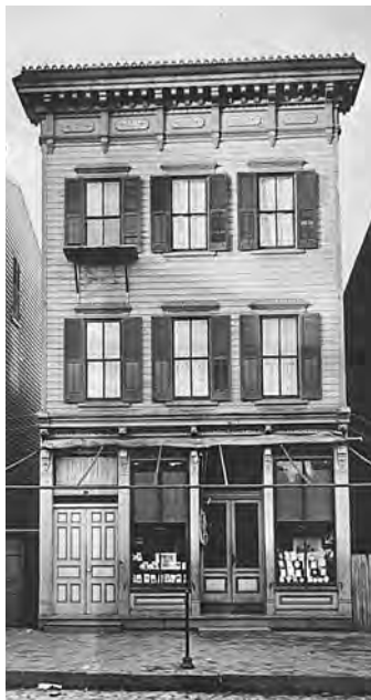
Figure 30. Italianate facade with bracketed cornice, 118 Main Street, 1888-95. During the second half of the nineteenth century, the vitality of commercial enterprise was expressed in the decoration of street facades. Bracketed cornices, door and window hoods, and elaborate storefronts embellished new and remodeled structures. (Marion Warren Collection, Maryland State Archives, MSA SC 985-112)
