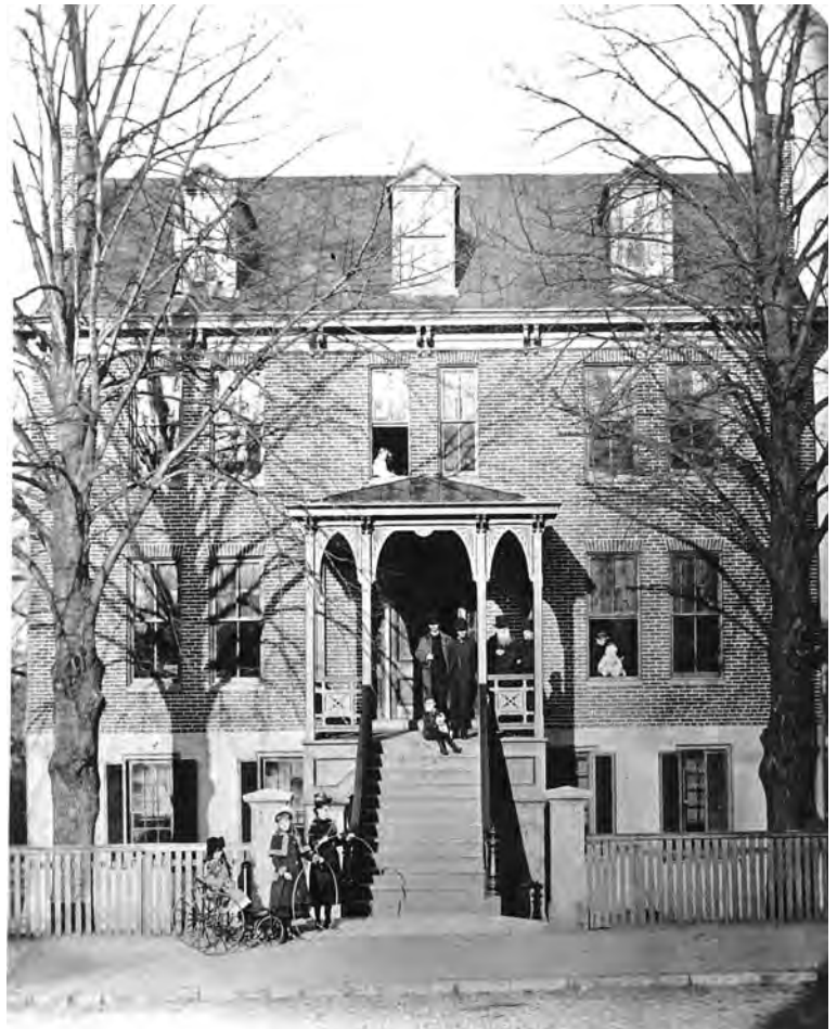
Figure 52. Calvert House, 58 State Circle, altered late nineteenth century. Paired windows separated by planar areas of brick work create a visually dynamic rhythm.
