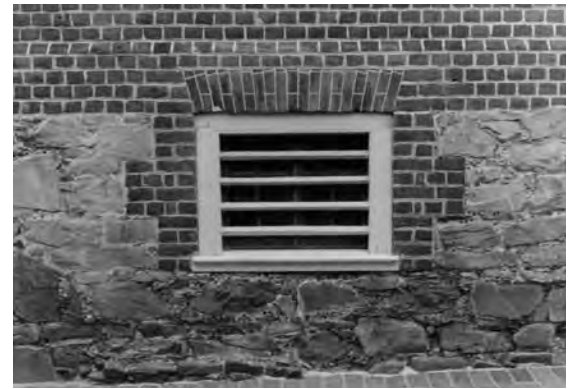
Figure 18 (above). Detail of galleting, William Paca House.
