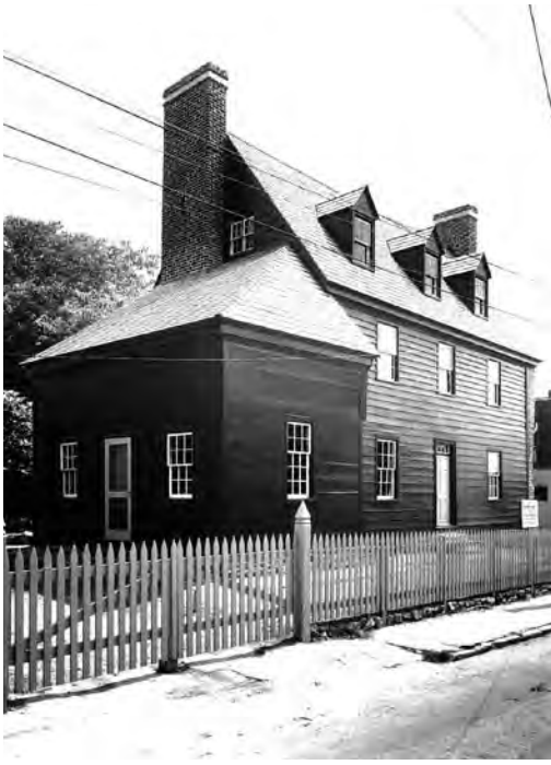
Figure 20. Shiplap House, 18 Pinkney Street, c. 1715. The steep roof, mix of three types of siding, small windows, and single pile floor plan are characteristic of early eighteenth century vernacular dwellings in Annapolis. (Marion Warren Collection, Maryland State Archives, MSA SC 1890-243)
