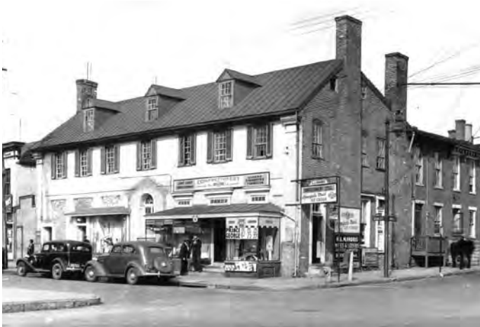
Figure 73. Historical photographs such as this view of Middleton Tavern, 2 Market Space, provide invaluable information regarding the earlier appearance of historic buildings. (Courtesy of Historic American Buildings Survey, Library of Congress. E. Pickering, 1936)
