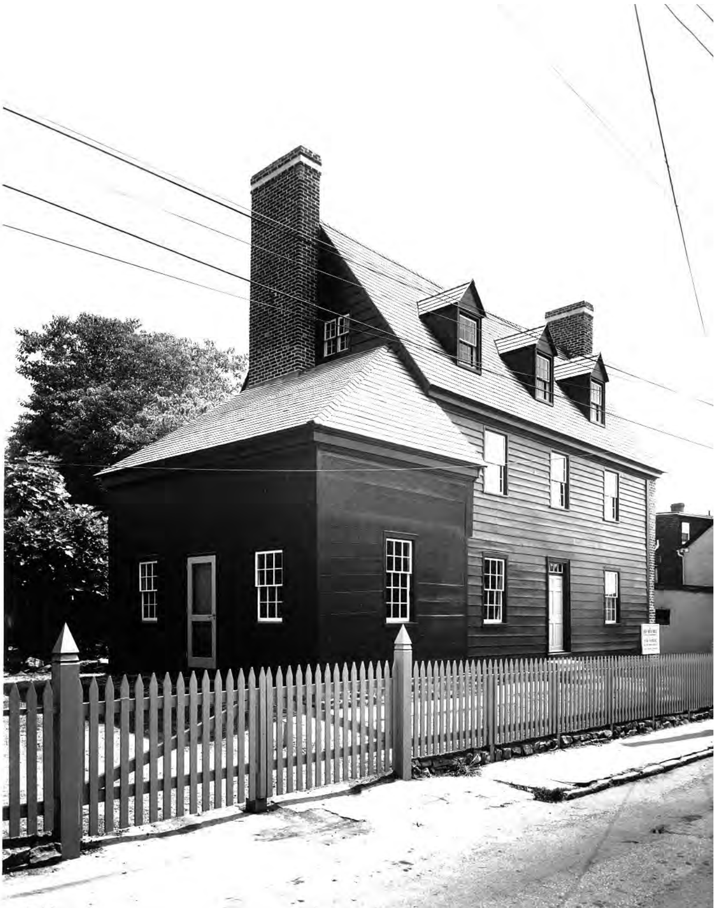
Figure 98. Shiplap House, 18 Pinkney Street. Its present appearance is a result of restoration efforts conducted in the 1960s and 1970s by Historic Annapolis Foundation. Today it serves as their headquarters. (Maryland State Archives Special Collections MSA SC 1890-243)
