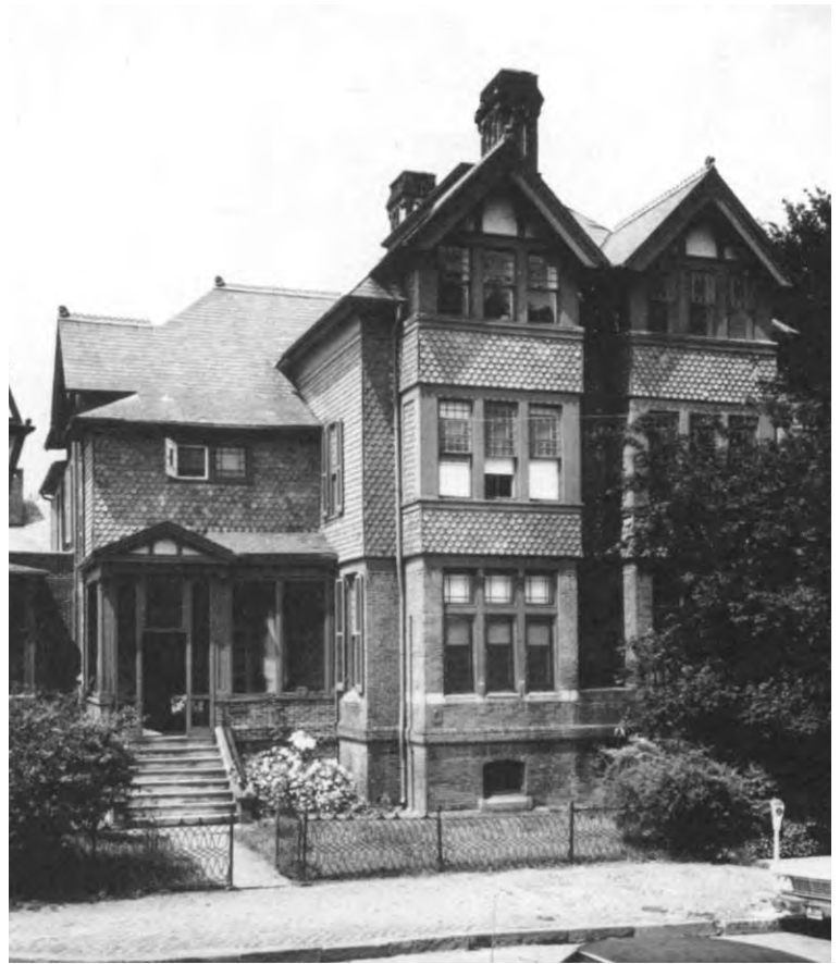
Figure 60. 86-88 State Circle, 1878. This pair of semi-detached dwellings skillfully employs the Queen Anne Revival use of projecting bays, paneled brick chimneys, specialized window shapes, and picturesque composition. (Marion Warren Collection, Maryland State Archives, MSA SC 1890-2897)
