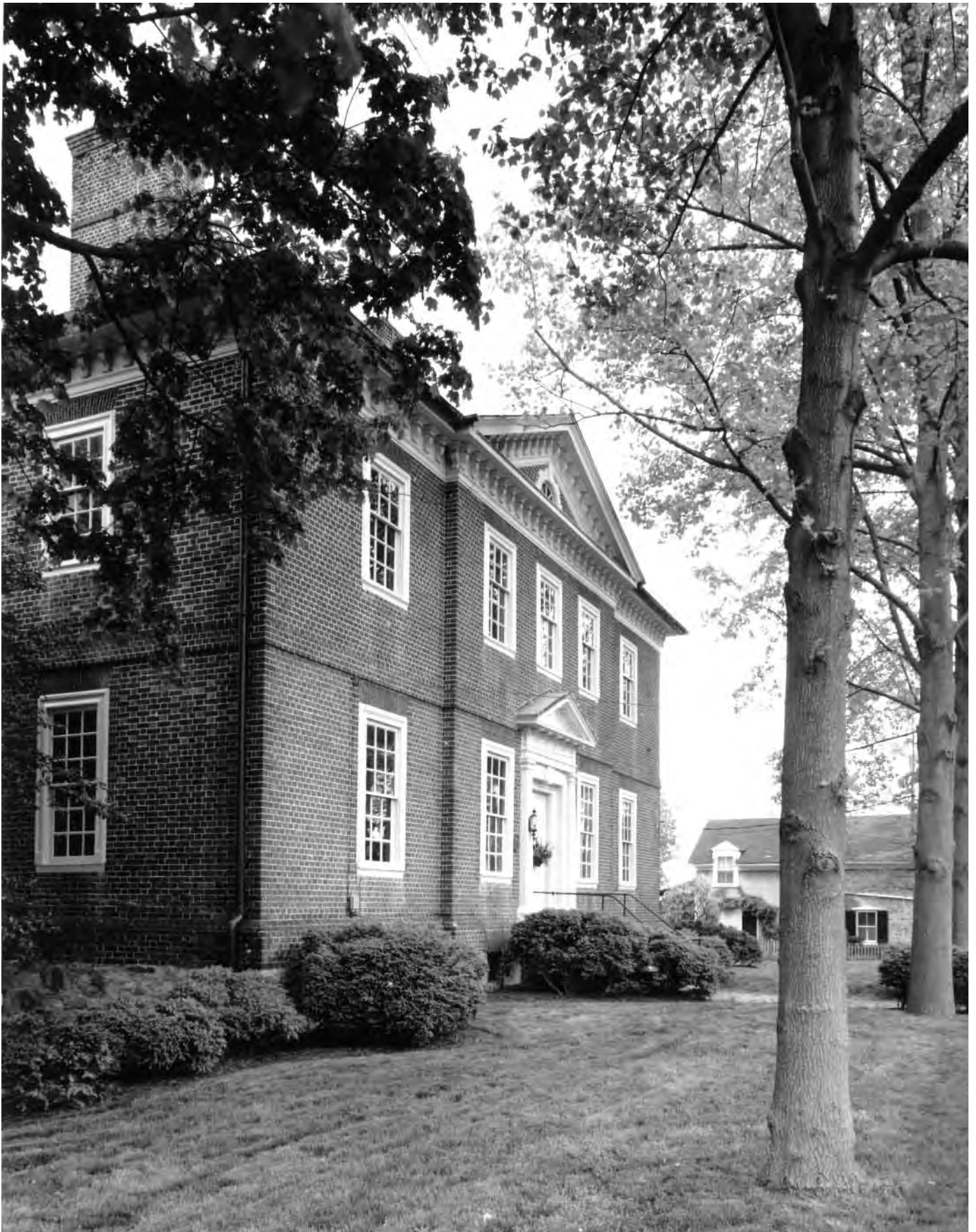
Figure 37. Upton Scott House, 4 Shipwright Street, 1762-63. The Upton Scott House was described as "the best town house in America" by Daniel Dulaney shortly after its completion. (Willie Graham, Colonial Williamsburg Foundation, 1996)
