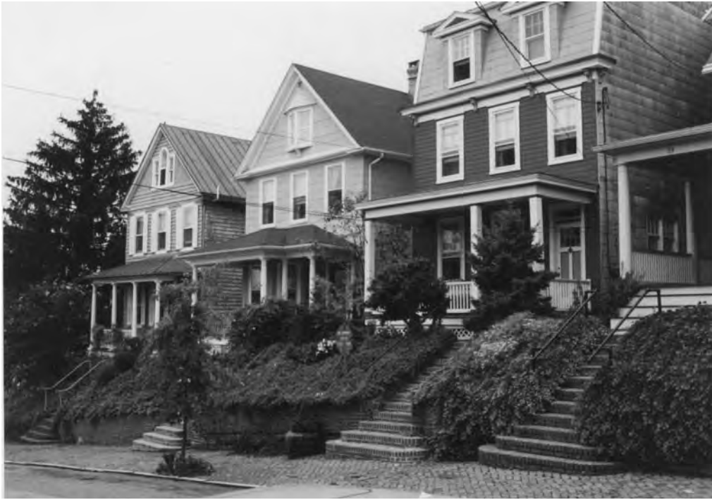
Figure 51. Houses along Market Street. The regular spacing of houses creates a rhythm along the street.
