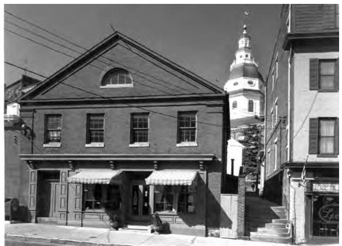
Figure 28. Greek Revival Commercial Building, 206 Main Street, about 1840. The temple form of the Greek Revival style is abstracted to a simple gable end with simple pilasters and lunette attic windows. (Marion Warren Collection, Maryland State Archives, MSA SC 1890-3506)
