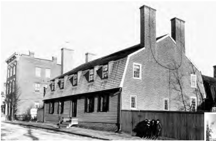
Figure 21 (above). Jonas Green House, 124 Charles Street, before 1735. This small scaled Georgian house portrays Georgian principles of symmetrical balance and horizontality. (Marion Warren Collection, Maryland State Archives, MSA SC 1890-244)
