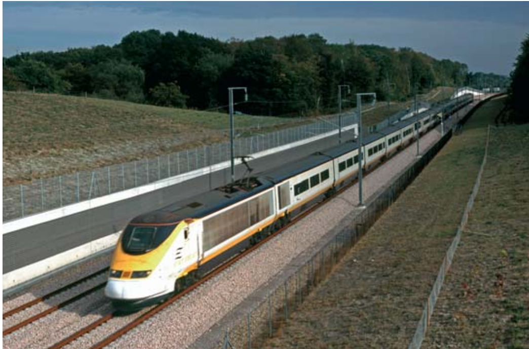
A Eurostar travelling on High Speed One, alongside sound insulating walls and embankments
