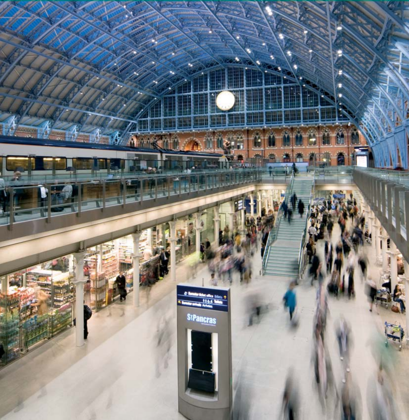
St Pancras Station, restored, expanded and reopened in 2007 as the terminus for High Speed One.
