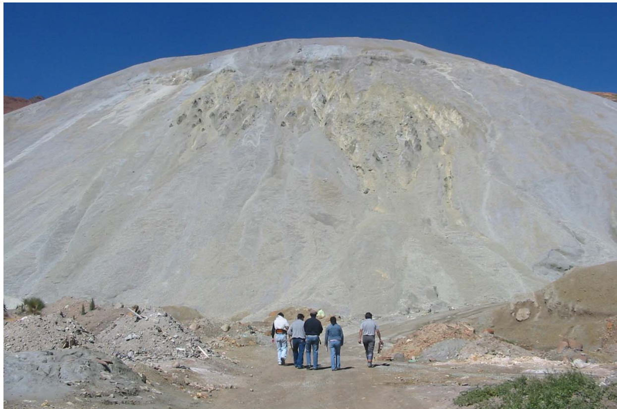
Figure 2: A portion of the Pailaviri tailings deposit which lies within the Huayna Mayu watershed. The Pailaviri tailings are less than 100m from Huayna Mayu, which drains to the Ribera de la Vera Cruz less than 2 km from the location pictured.
