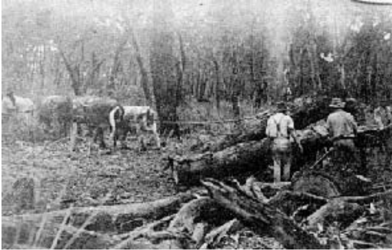
Plate 2.1 Stringy barks being harvested at Hindmarsh Tiers to be used to shore up BHP mines c1917 (newspaper clipping provided by Shirley Cushion, original source unknown)
