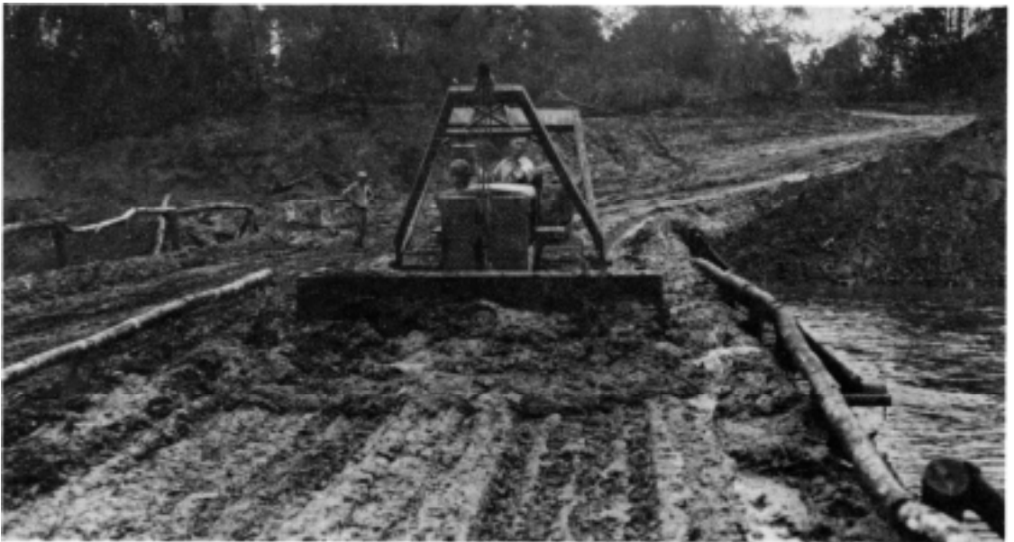
Engineers of the 1880th Engineer Aviation Battalion scrape the thick layer of mud caused by two days of rain from a temporary bridge near Myitkyina, Burma
