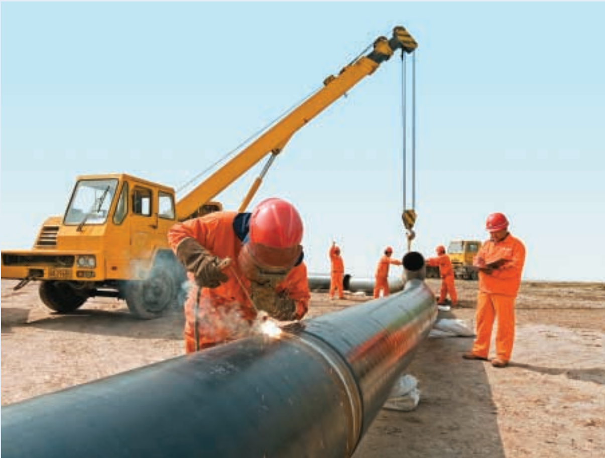
In a joint tri-partnership, Hong Kong and China Gas has participated to construct a high-pressure natural gas pipeline system in Hangzhou that will eventually supply household, commercial and industrial business customers.
