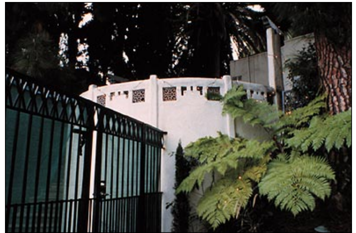
Retaining wall of the Ternary Gardens
