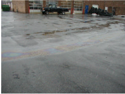
This parking lot borders and drains into a tributary of the Wallkill.
