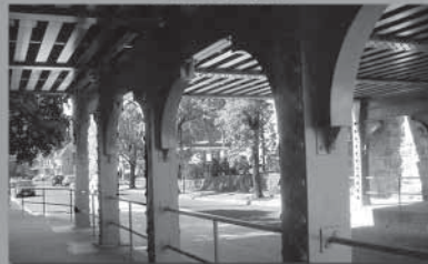
Grant Avenue Bridge Rehabilitation Plainfield, NJ
