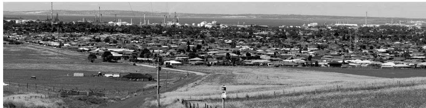
The Bypass follows the freeway reservation which has been in place for more than 20 years on Geelong's western outskirts
