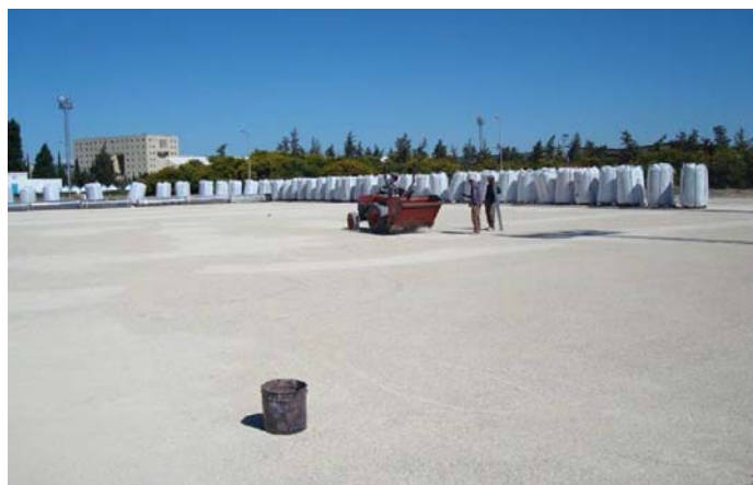
Preparation of the ground.
