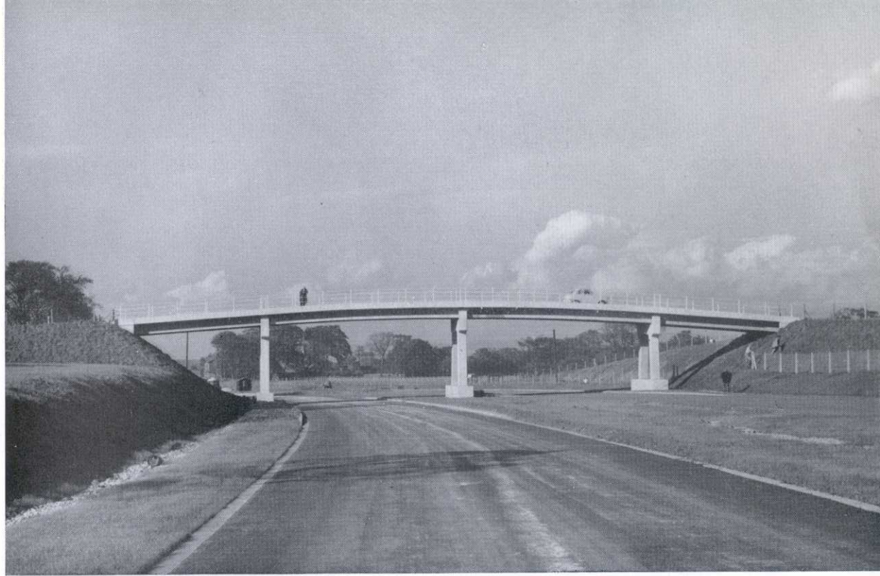
PLATE I. LANE END FARM OCCUPATION BRIDGE.
