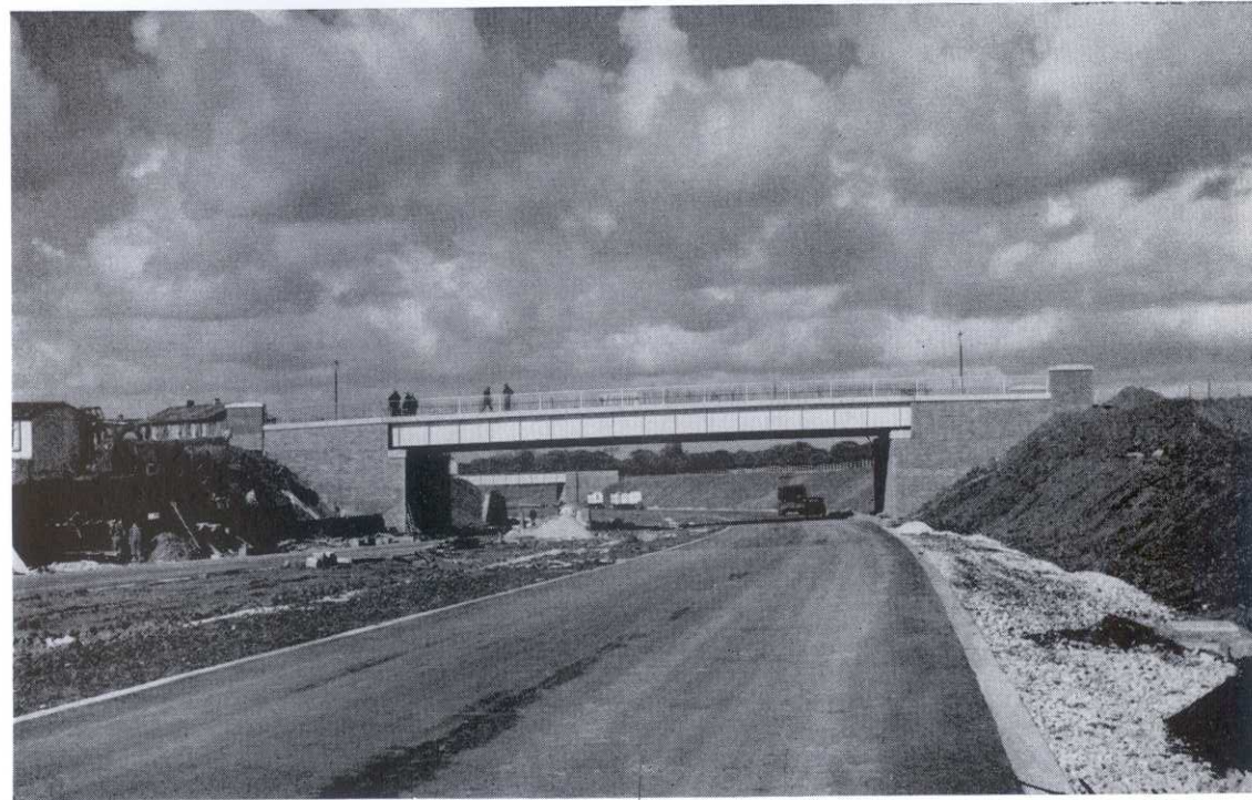
PLATE 7. LONGRIDGE ROAD BRIDGE.
