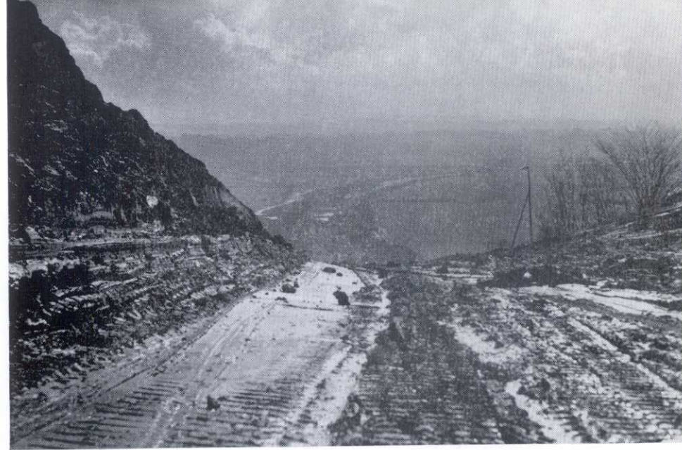
PLATE 5. NORTH ESCARPMENT TO RIBBLE VALLEY UNDER CONSTRUCTION.
