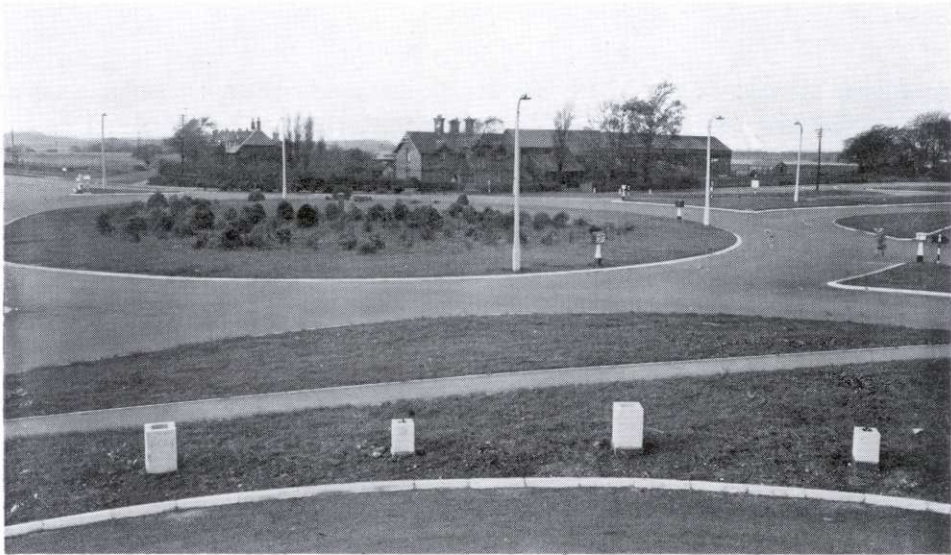
RECONSTRUCTED ROUNDABOUT AT JUNCTION WITH LIVERPOOL—EAST LANCASHIRE ROAD AT WINDLE. COMMENCEMENT OF NEW ROAD SHOWN ON RIGHT
