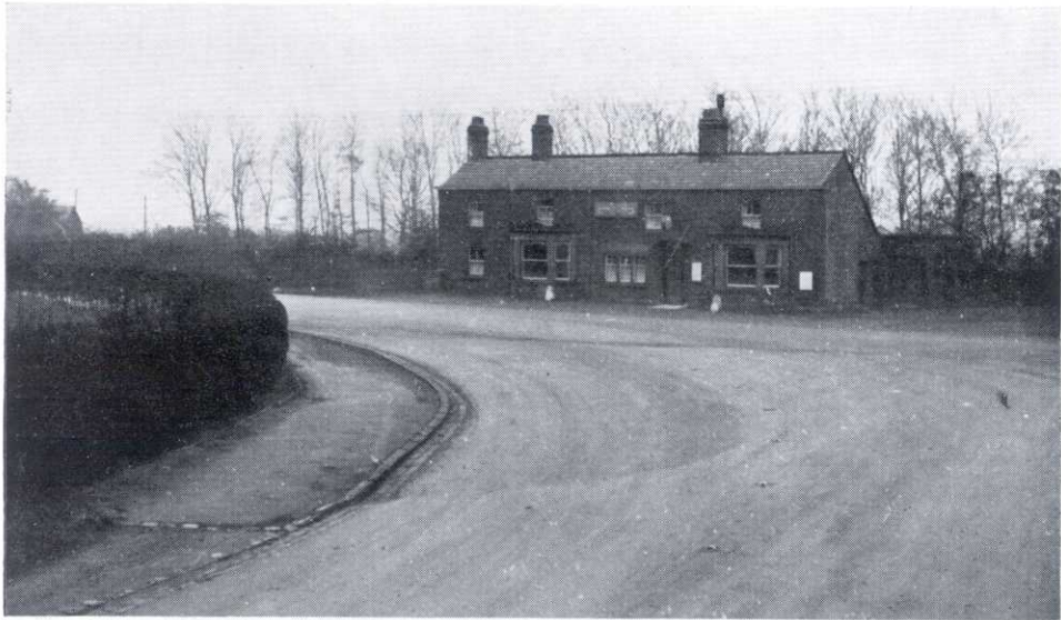
VIEW OF OLD ROAD SHOWING RIGHT-ANGLE BEND AT TOP OF BOTTLE AND GLASS BROW
