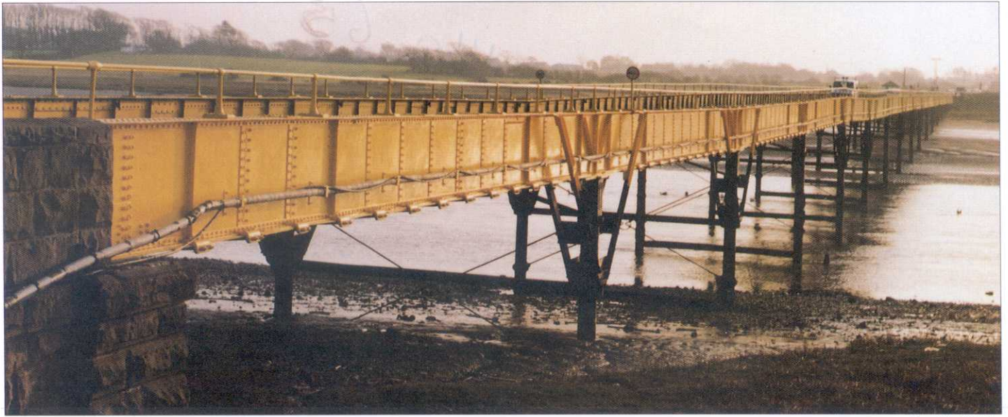
Shard Toll Bridge
