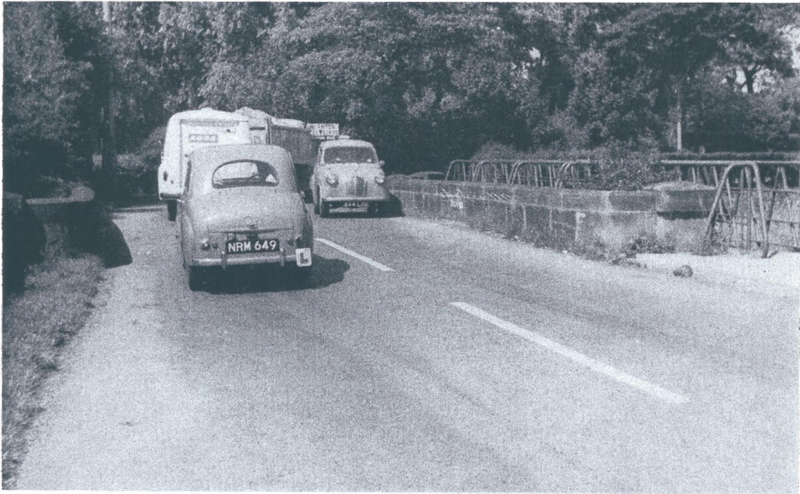
PLATE 26.—Kirkham-Fleetwood Road A585.—Skippool Bridge.
