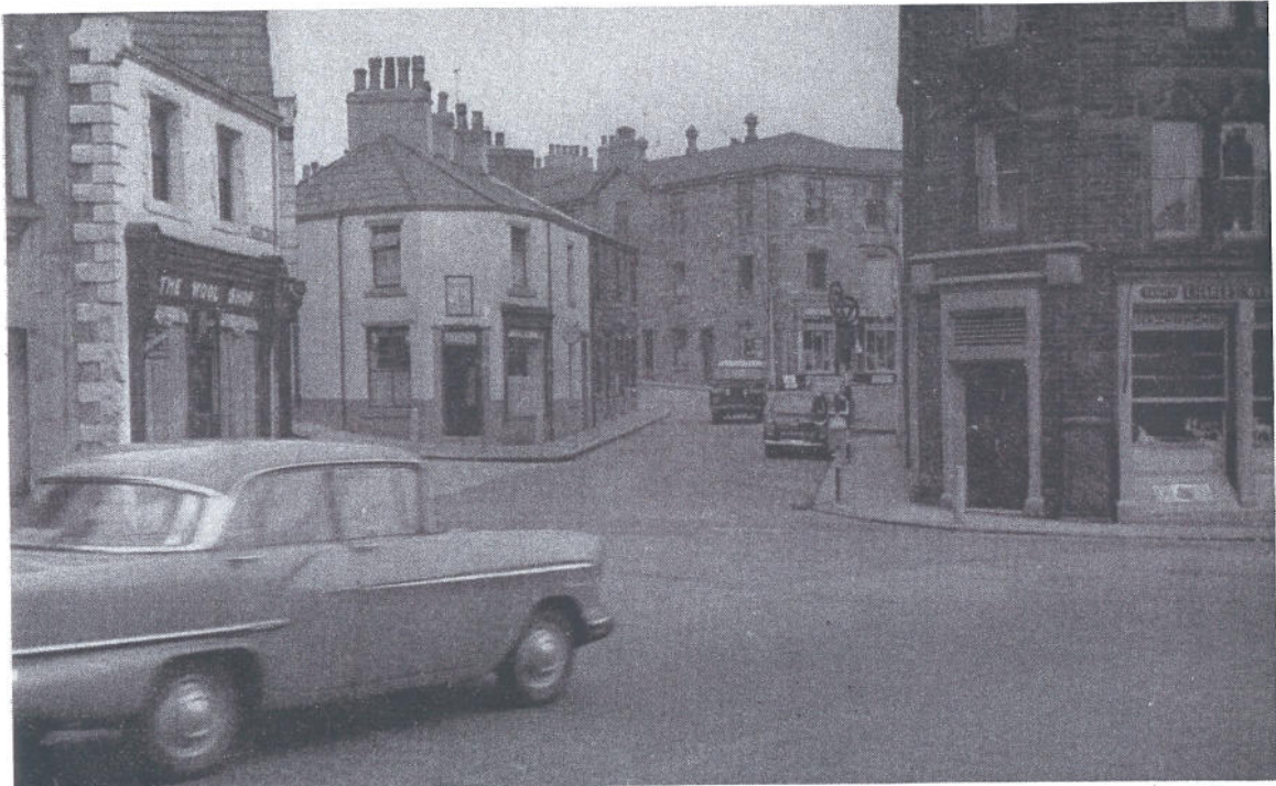
PLATE 31.—Junction of A671 and Moor Lane B6247, Padiham.
