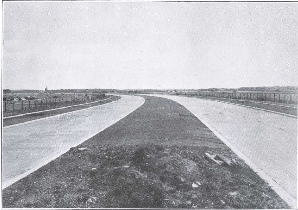
View from Alt Bridge looking south. Construction in progress.
