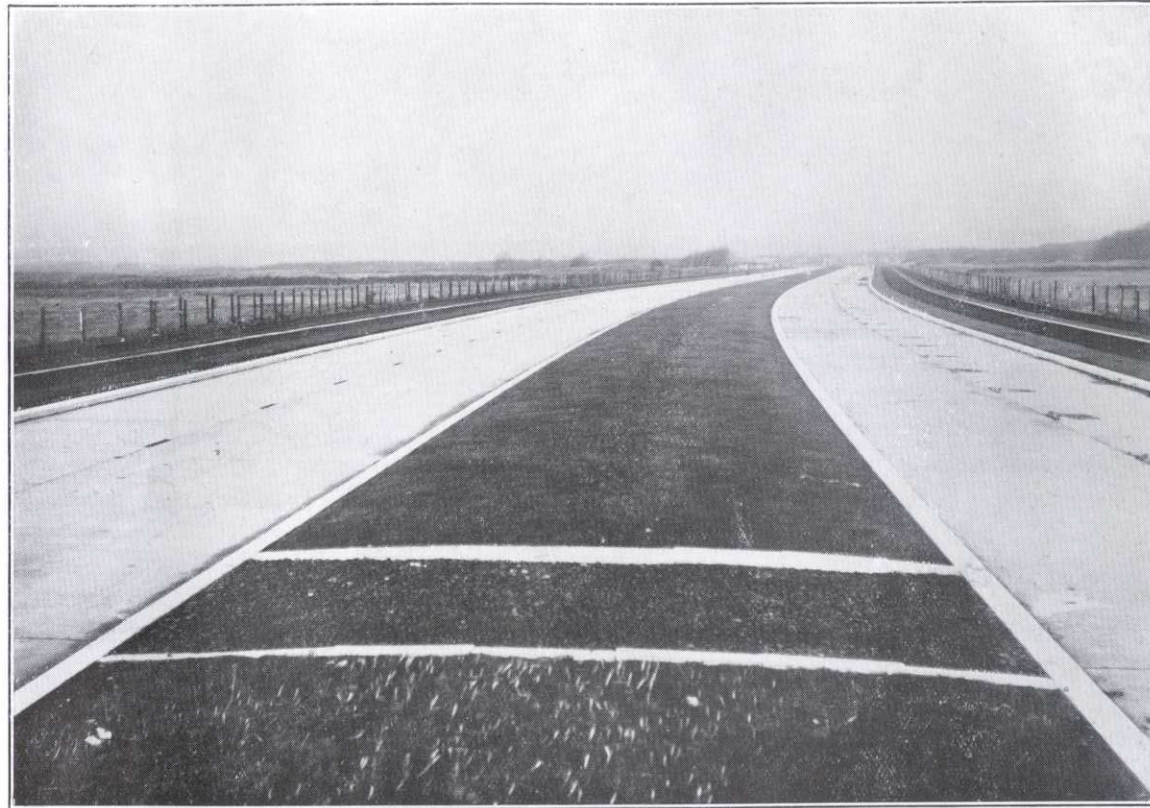
Road (in course of construction), showing northerly portion of the By-pass.
