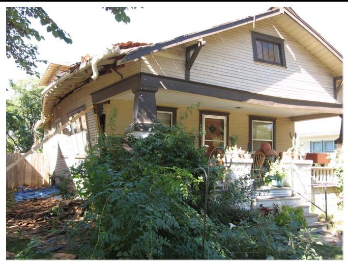
Engine 10 and Squad 1 were sent to an assist a citizen call, on our arrival this is what we encountered! The roof was overloaded and began to collapse as the roofers were tearing off shingles. The roofers quickly exited the roof and propped a 2x4 against the load bearing wall on the South side of the structure.
