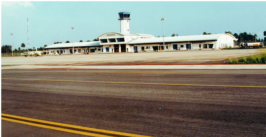
The old airstrip (above) and the new (below)
