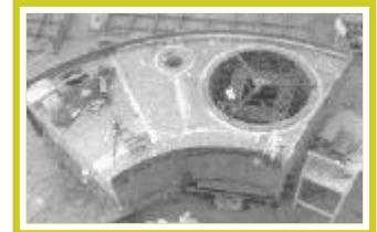
Roof Slab Sector
