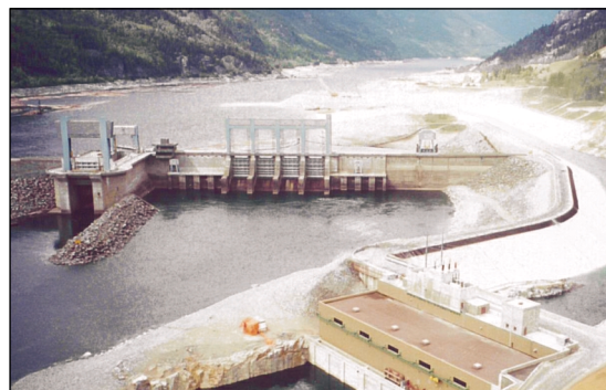
The 185 MW Arrow Lakes project, under construction on the Columbia river.
