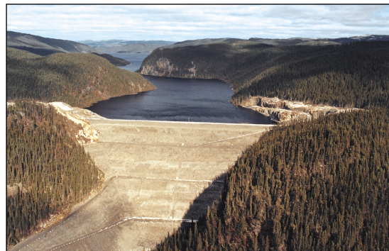
The 171 m-high rockfill dam at the Ste-Marguerite 3 plant, recently completed in Québec.
