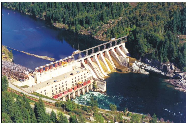
The 43 m-high Brilliant dam and powerplant on the Kootenay river, BC.
