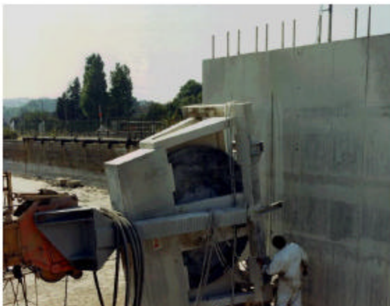
Fig. 8. Removal of Active Concrete
