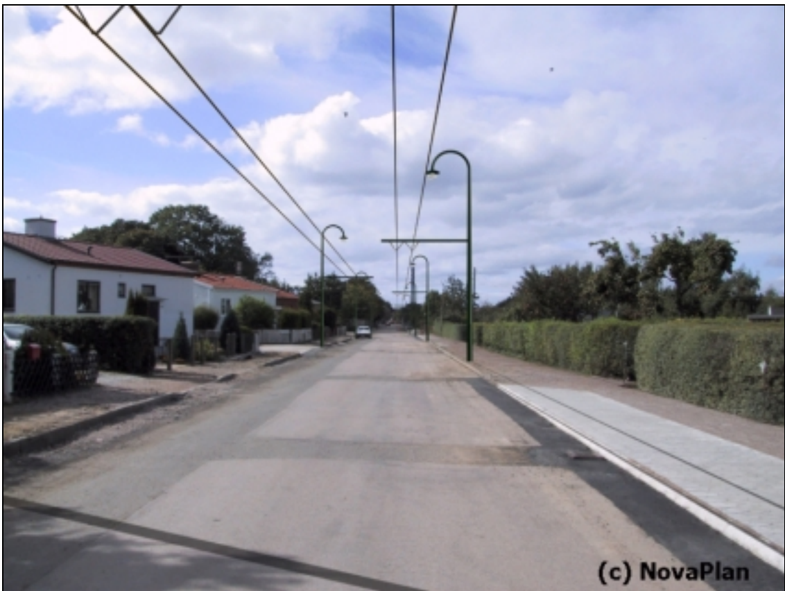
Example of the studied poles for the overhead wire
